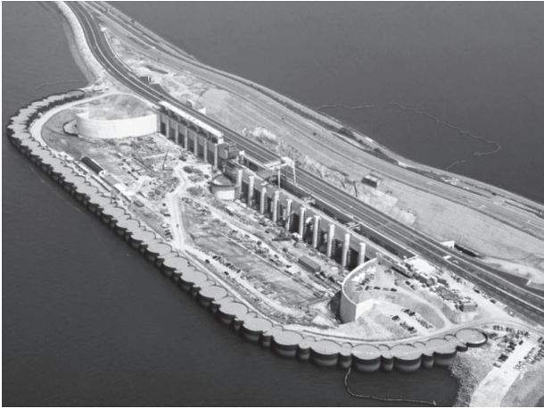
Figura 7 – Sihwa Lake Tidal Power Station, Coreia do Sul
